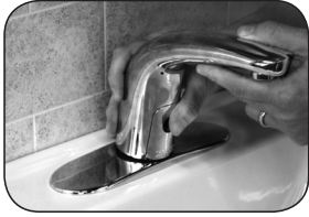
11. Re-install Faucet. Secure faucet to sink.
