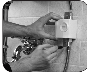
3. Mark holes. Position mounting bracket and mark mounting holes.
