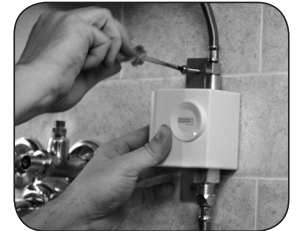
5. Secure SSPS to wall. Insert anchors into holes and mount SSPS unit to wall with supplied screws.
