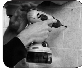
4. Drill holes. Drill holes for screw anchors.
