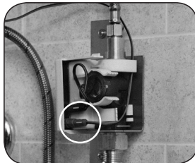
7. Connect wiring. Remove cover and connect green power adapter wire to green power receptacle inside SSPS and secure into wire harness.
